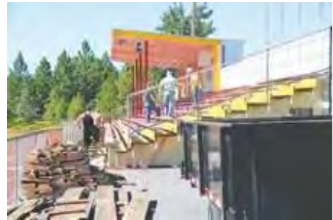
Daily Recovery Center workers replace old bleacher boards Wednesday at Miner Stadium. Daily News Photo/Kevin Dickinson
