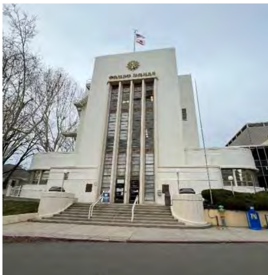
Figure 8. Primary (south) façade, view north, showing the courthouse building following 1937 alterations, including symmetrical façade arrangement, fenestration pattern and material, and ornament including lettering, clock, and flagpole (ARG, 2022)
