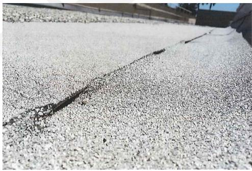
**Above**: Previous roof in need of repairs **Below**: Newly repaired roof with reinforced acrylic coating
