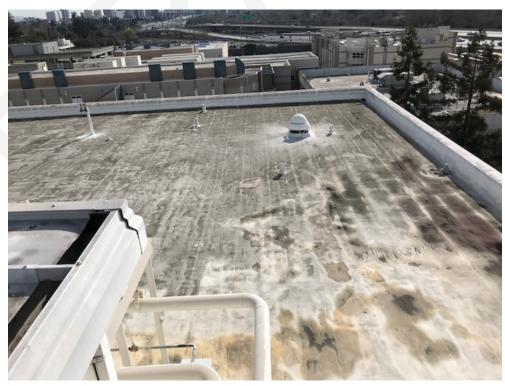
**Above**: Old roofing material (brown) compared to new roofing material (white) **Below**: Newly replaced roof
