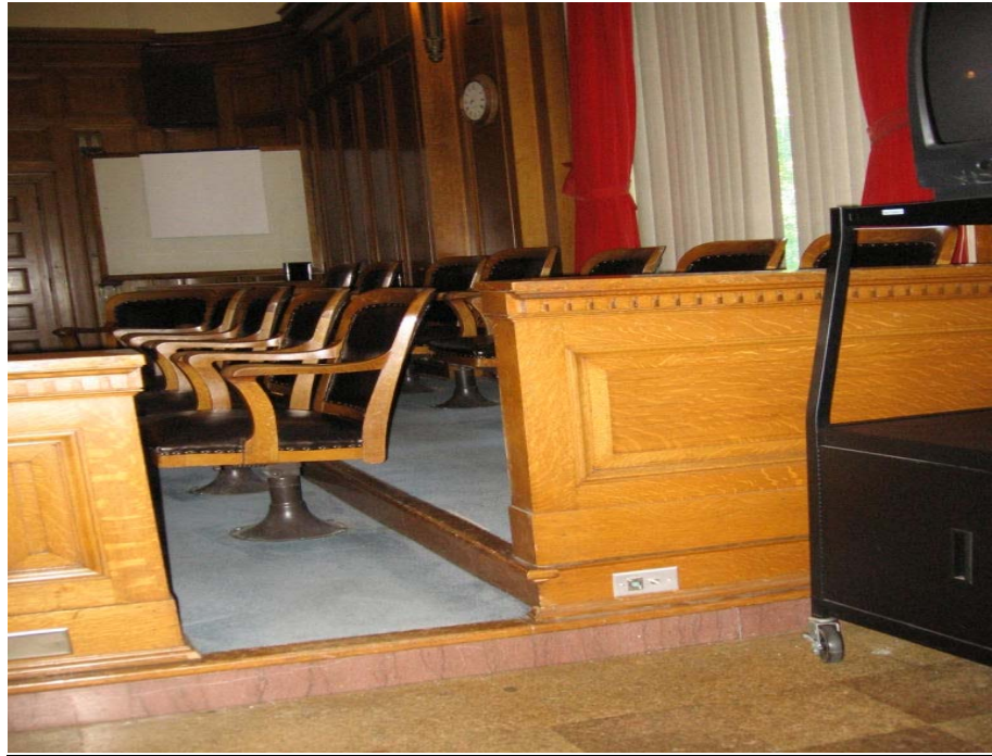
FIGURE 2.7.d Witness Stand Does Not Comply with Current ADA Standards
