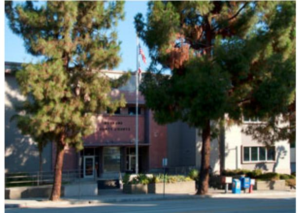
The main portion of the building was constructed in 1953, and an addition was constructed in 1994. The 1953 portion of the building is a wood structure with wood and steel joists and steel beams supporting slightly pitched metal decks covered with single-ply TPO roofing. The 1994 addition is CMU with portions exposed and portions covered with ceramic tile, and a flat single-ply TPO roofing system. Although connected, the two building elements have independent HVAC systems.
