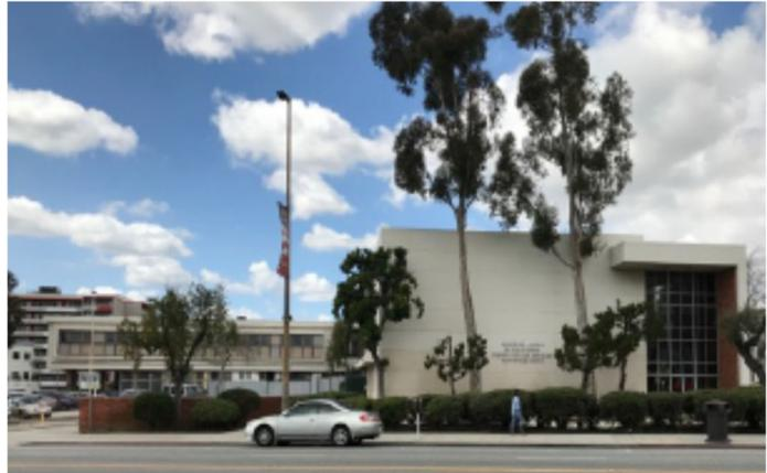
The structure includes a basement and three above-ground levels (main, second, and penthouse). The building was constructed of load bearing cast-in-place concrete with concrete masonry unit (CMU) exterior walls.
