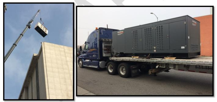
**Before**: Removal of the old generator. The unit weighed over 21,000 lb., approximately twice as much as the new generator (*above left*).
