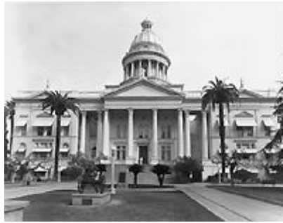
Hailed as "the grandest and noblest edifice that has ever been planned and contemplated in this valley," Fresno's courthouse could barely keep up with the county's booming population.
